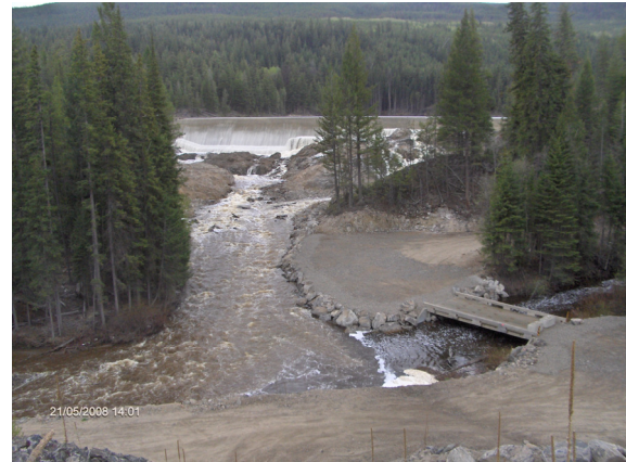
Spillway at Thirsk Dam flowing
