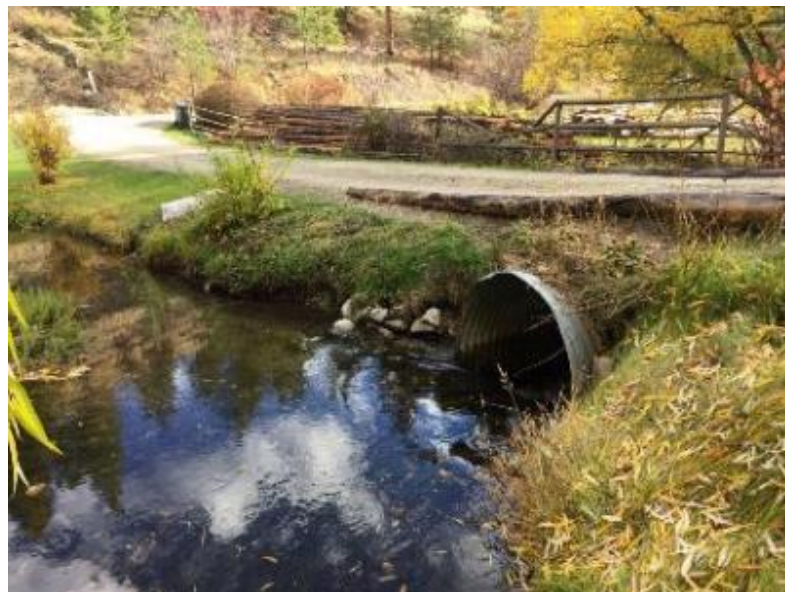
Figure – Culvert Inlet
