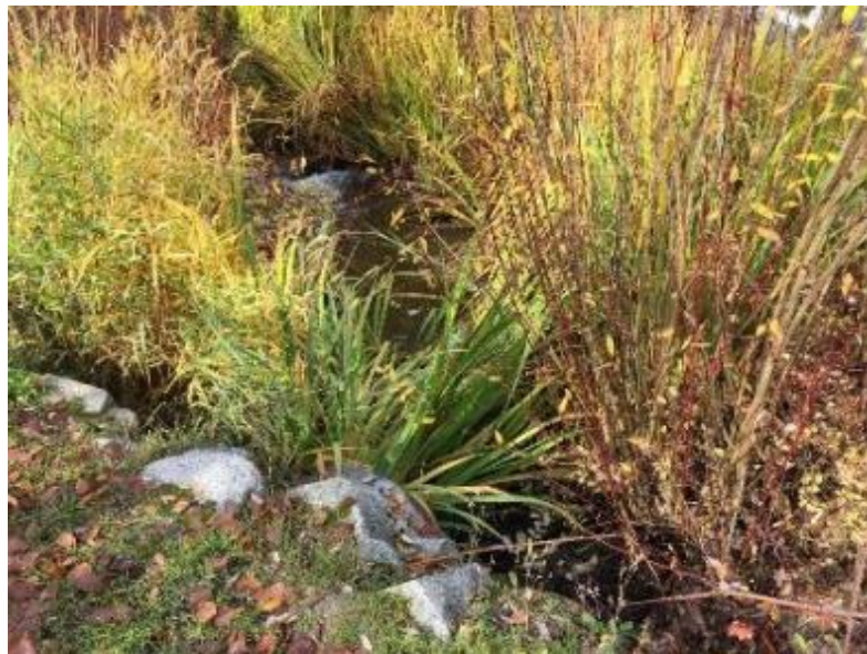
Figure – Culvert Inlet
