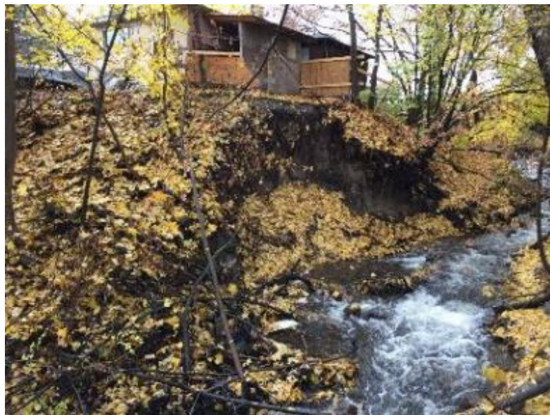
Figure – Slope Failure
