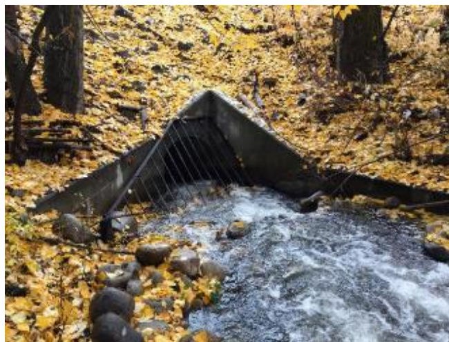
Figure – Culvert under Hwy 97 Inlet
