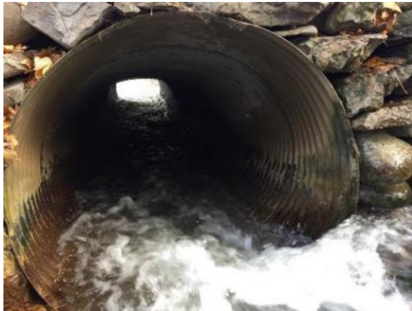
Figure – Pohlman Road Culvert
