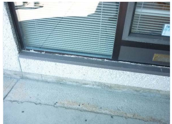
Photo Env17 Windows
