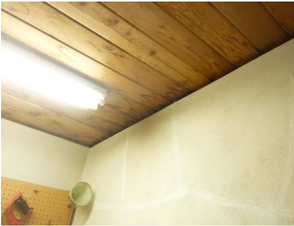
Photo Env25 Attic Space
