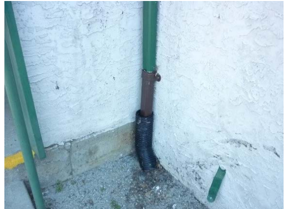
Photo Env15 Perimeter Drains
