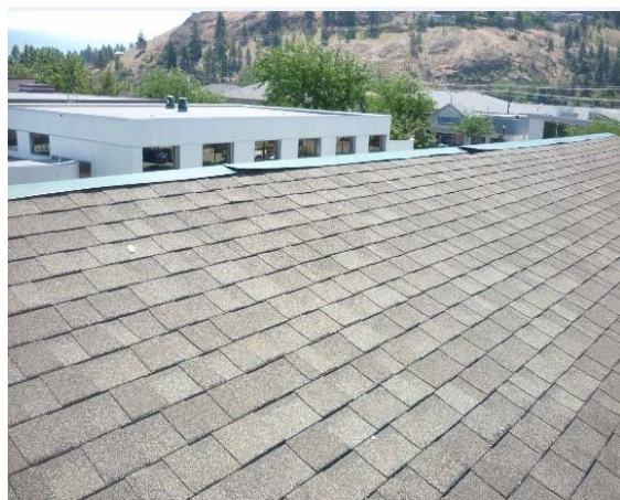
Photo Env11 Roof Flashing
