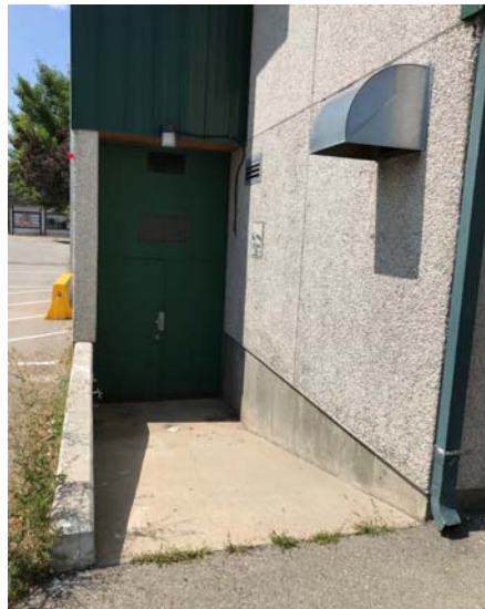
Photo A12 View of South mechanical room exterior door.
