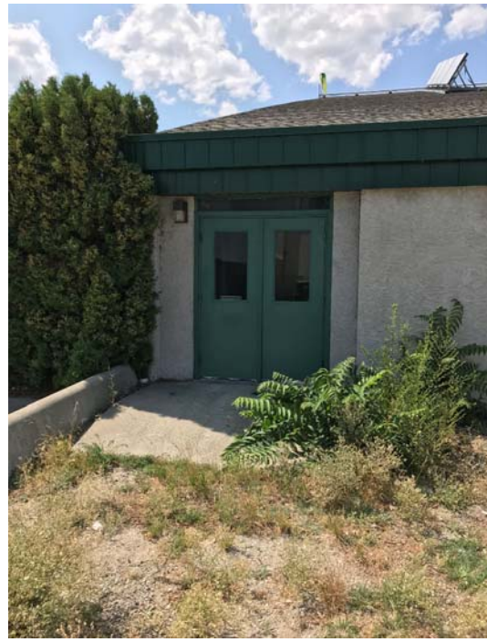
Photo A16 Exterior view of South-East pool exit doors.
