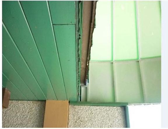
Photo Env19 Soffit and Fascia
