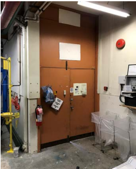
Photo A11 View of South mechanical room exterior door.
