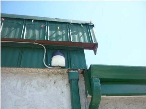
Photo Env14 Gutters and Downspouts
