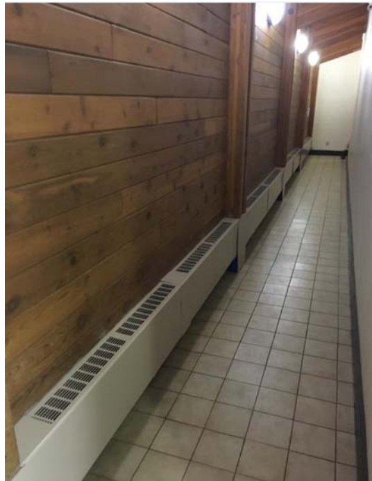
Photo M4 Radiation Wall Fin
