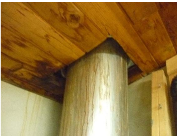
Photo Env10 Roof Penetrations
