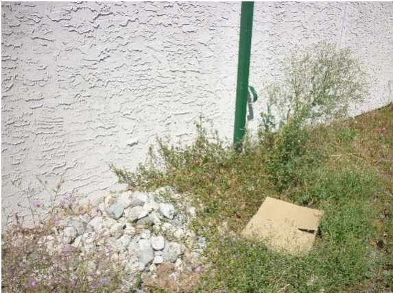
Photo Env6 Stucco Cladding
