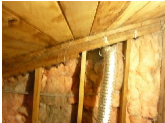
Photo Env7 Wall Penetrations
