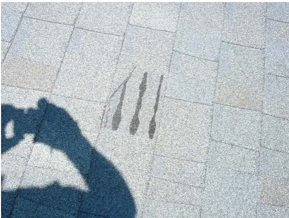
Photo Env8 Roof Shingles
