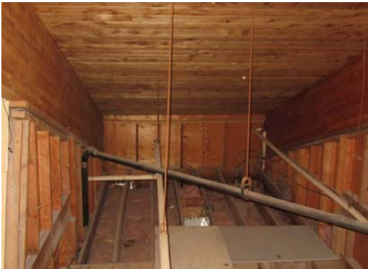
Photo S5 Framed ceiling now serves as mechanical service mezzanine.
