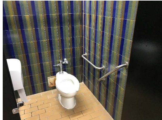
Photo A22 View of typical barrier free water closet in pool area.
