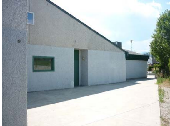
Photo Env1 North Building Elevation
