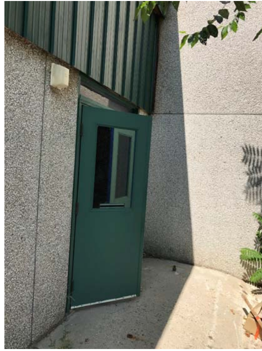
Photo A14 Exterior view of South pool exit doors.
