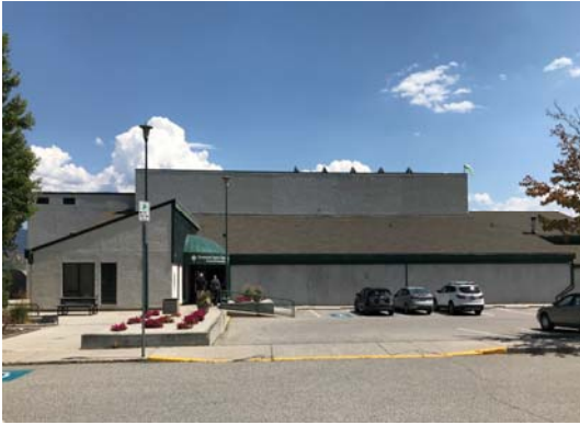
Photo S1 View of West elevation and main entrance.
