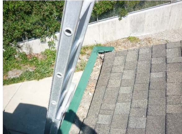
Photo Env13 Gutters and Downspouts
