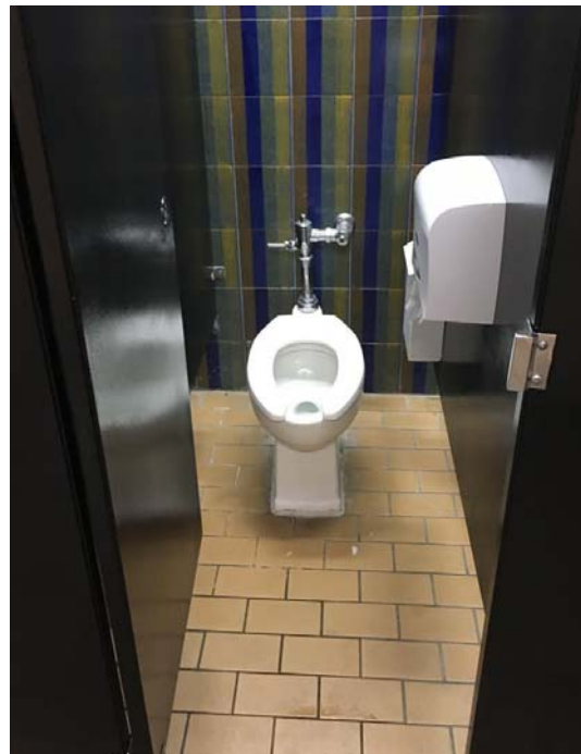
Photo M8 Typical Water Closet
