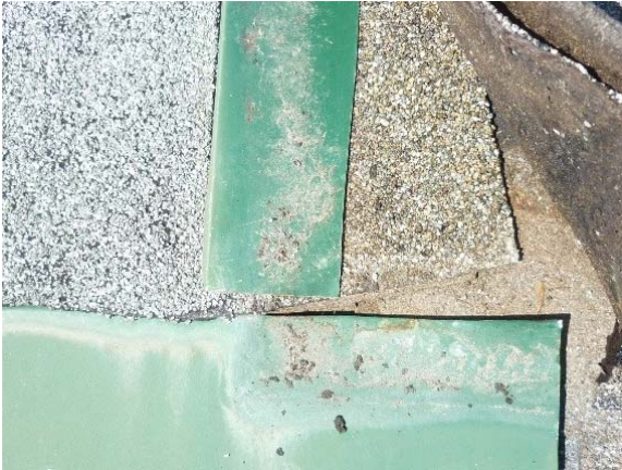
Photo Env12 Roof Flashing
