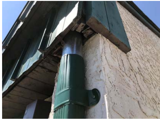
Photo A10 View of typical soffit to downspout condition.
