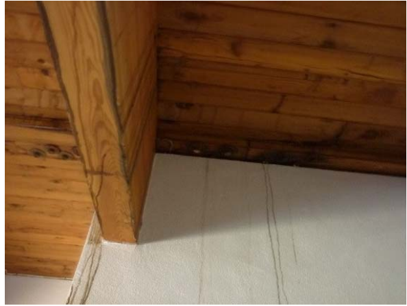
Photo Env24 (photo provided by District) Pool Area to mezzanine wall
