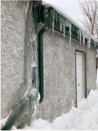
Photo Env23a (photo provided by District) Storage Shed
