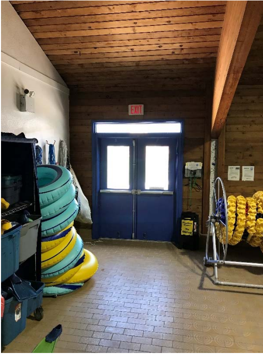
Photo A17 Interior view of North-East pool exit doors.
