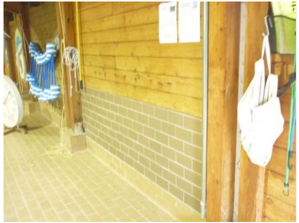
Photo Env26 Pool Deck Perimeter Walls
