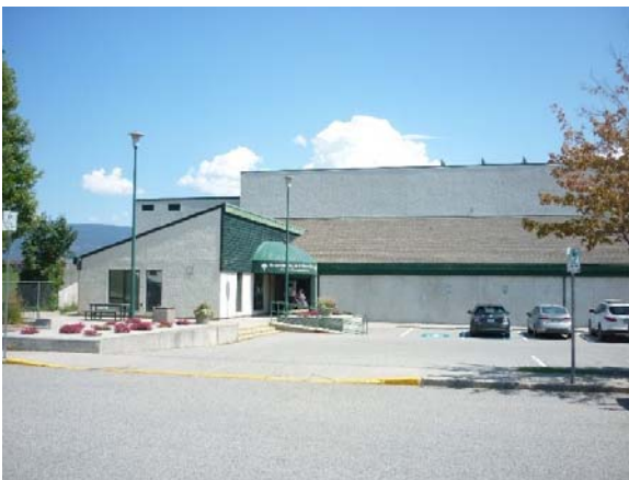
Photo Env4 West Building Elevation
