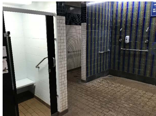
Photo A24 View of grab bars installed in change rooms.
