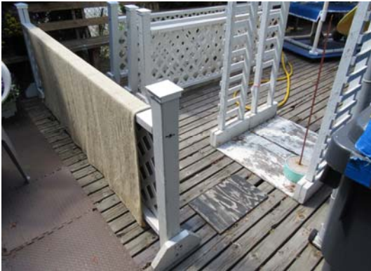
Photo S9 Exterior Deck
