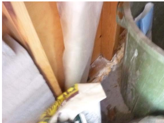
Photo Env23 (photo provided by District) Storage Shed
