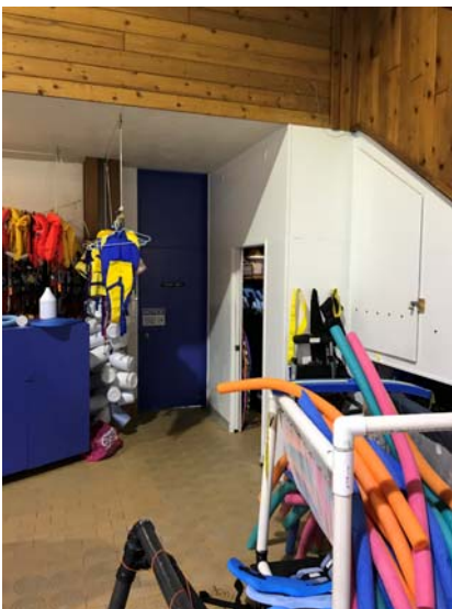
Photo A25 View of equipment room added under stairs.
