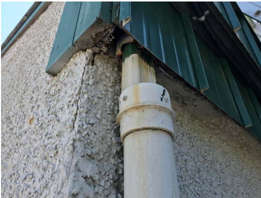
Photo A9 View of typical soffit to downspout condition.
