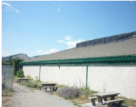
Photo Env3 East Building Elevation
