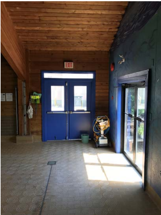
Photo A15 Interior view of South-East pool exit doors.
