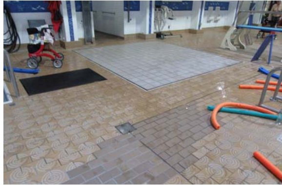
Photo S2 View of pool deck tiles
