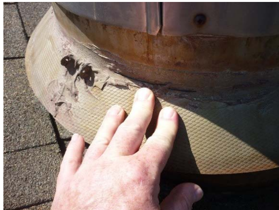
Photo Env9 Roof Penetrations
