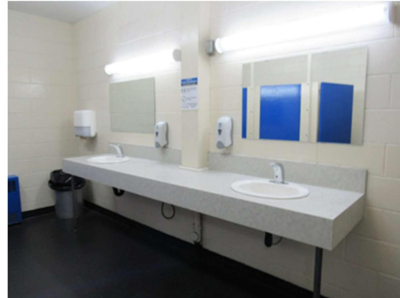
Photo #A16: Typical interior finishes of washroom in main floor.
