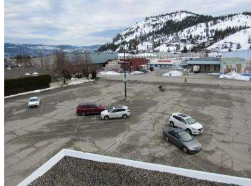
Photo #A2: Current condition of the parking stall marking.
