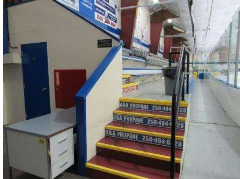
Photo #A12: Interior finishes of corridor inside of Rink.
