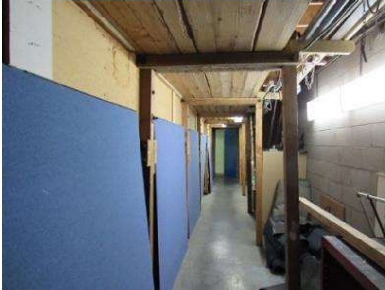
Photo #A17: Storage under bleacher area after a fire. All storage areas should be covered by Gypsum Board.
