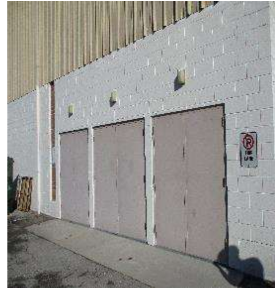
Photo #E16: Roof mounted LED lights installed in every elevation of the building.
