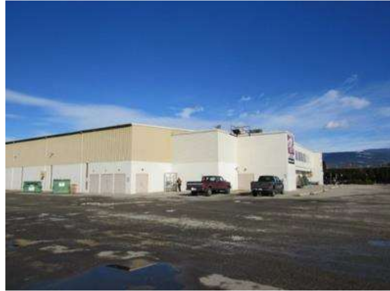
Photo #A4: Exterior cladding, windows, door - southwest elevation.
