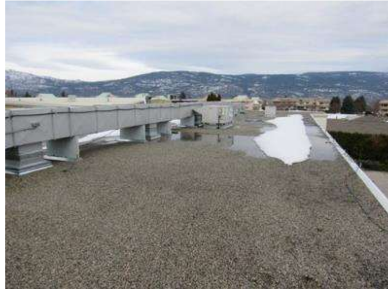
Photo #A24: Flat roof with BUR.
