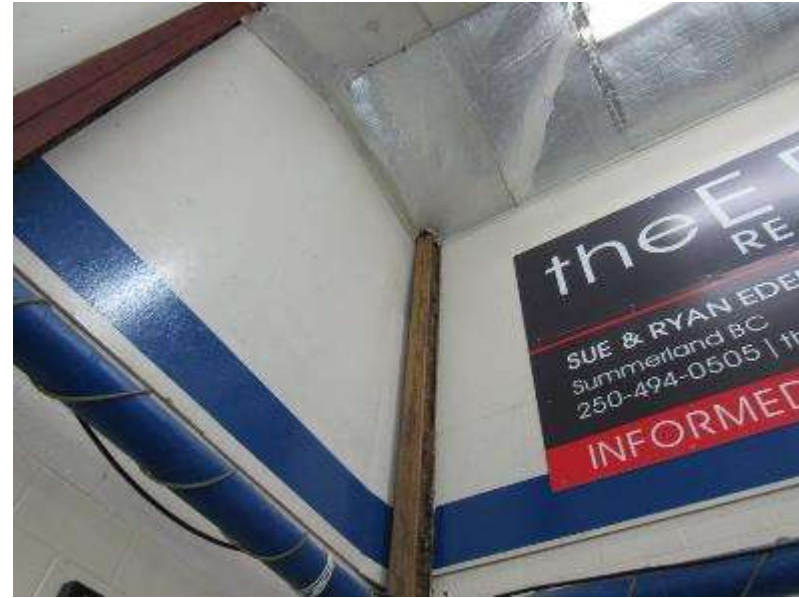
Photo #S10: Exterior Steel columns.
