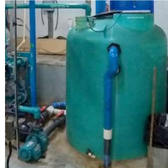
Photo #M30: Condenser Water Tank.
