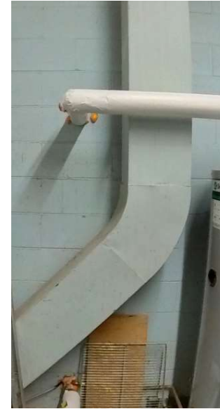
Photo #M28: Concession Range Welded Ductwork up to roof. No Access doors available.
