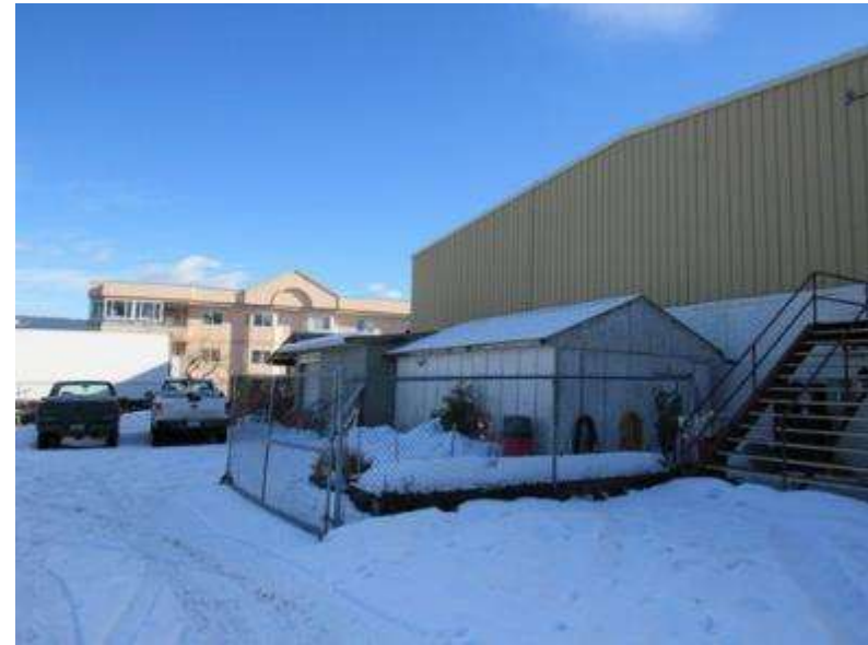
Photo #A8: Ancillary Building and Chain rink fence and Hockey Rink egress stair.
