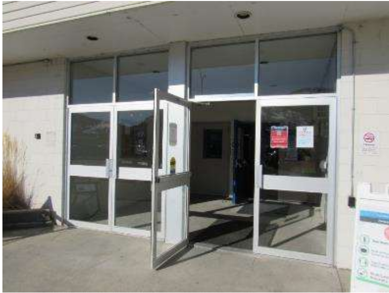
Photo #A9: Main Entrance Doors.
