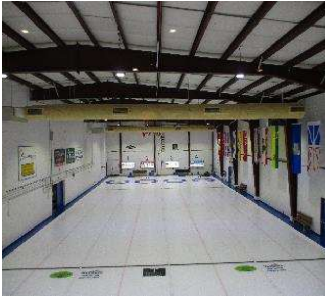
Photo #E13: Curling rink suspended LED lighting.
