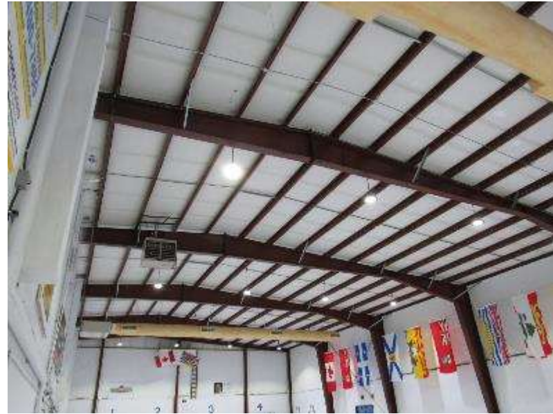
Photo #S2: Curling rink roof steel structure.
