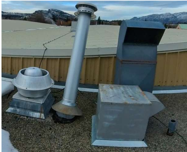
Photo #M29: Typical Exhaust Fans (Upblast - for Ranges, Square box - for Washrooms & Lounges) & Make-up Air Ductwork.
