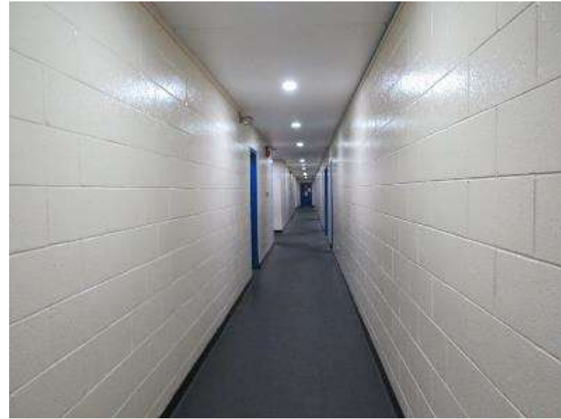
Photo #S8: CMU structural walls.
