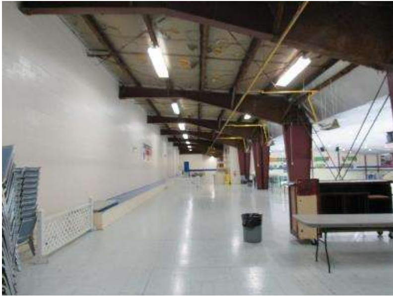
Photo #S1: Ice arena roof steel structure.
