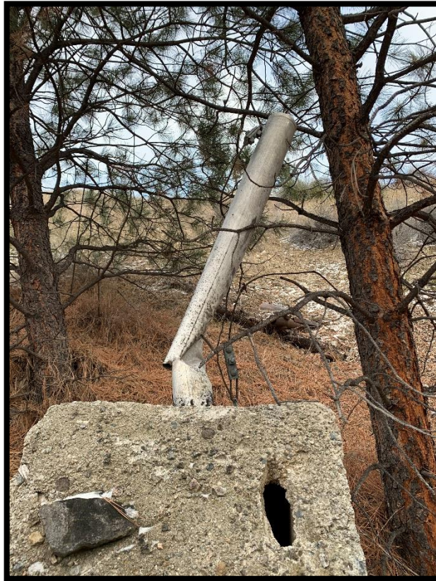
Photo 7: View of a lead pipe and concrete block found on site.
