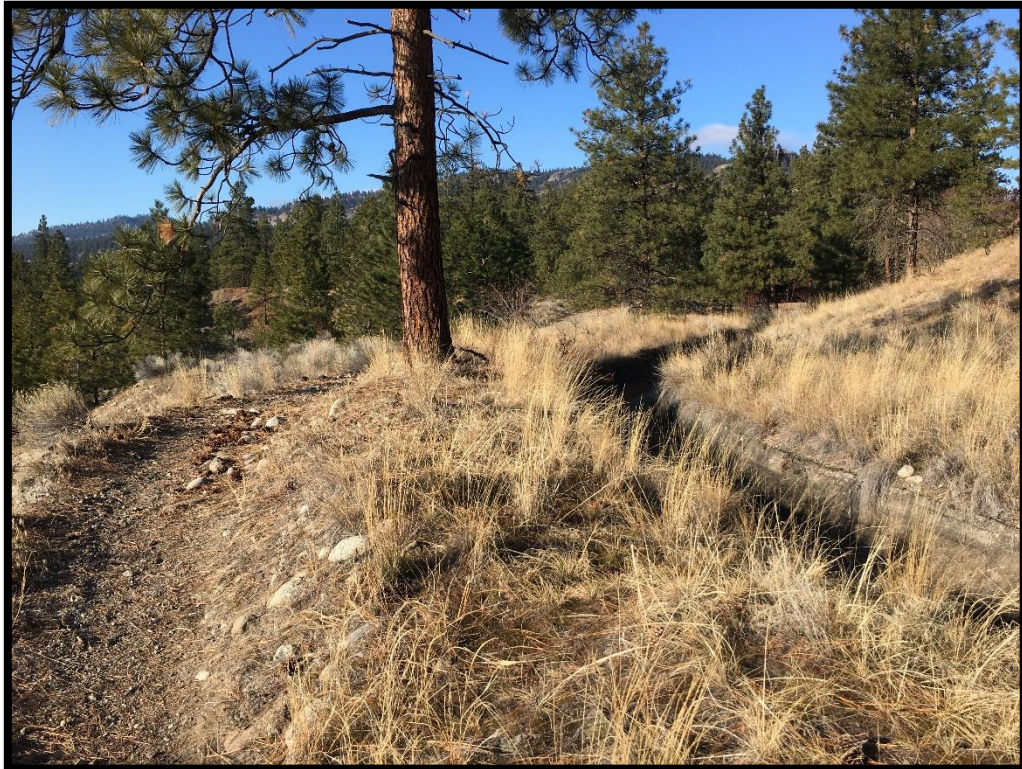
Photo 10: View of the concrete irrigation flume and hiking trail that runs along the north portion of the site.
