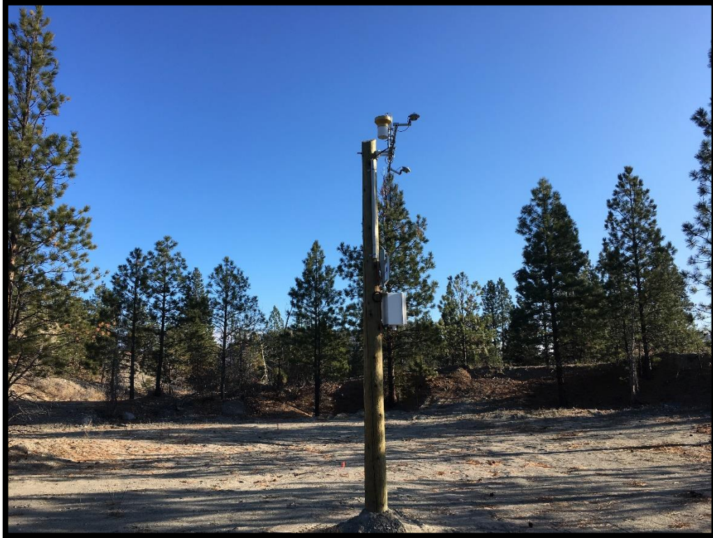
Photo 13: A view of the potential solar monitoring station location, looking east.
