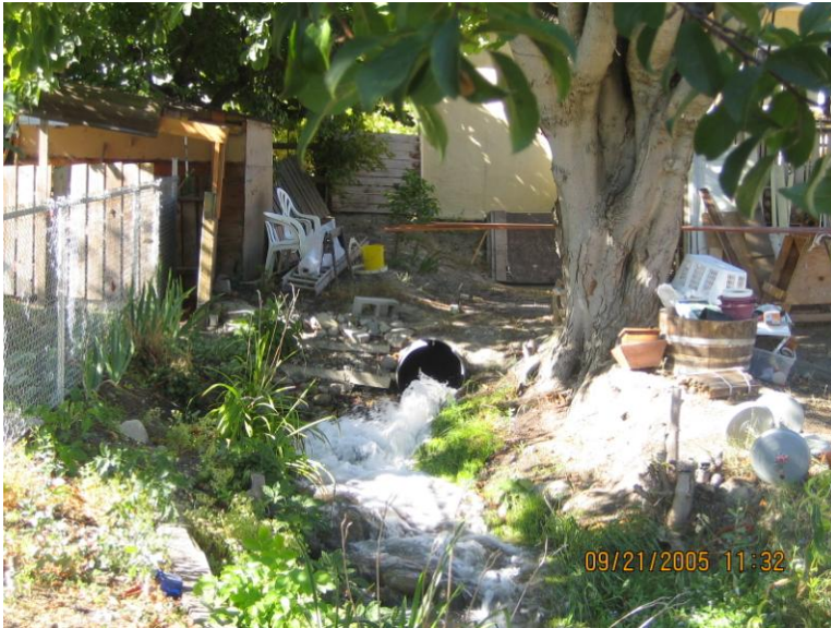
West side – Looking West
