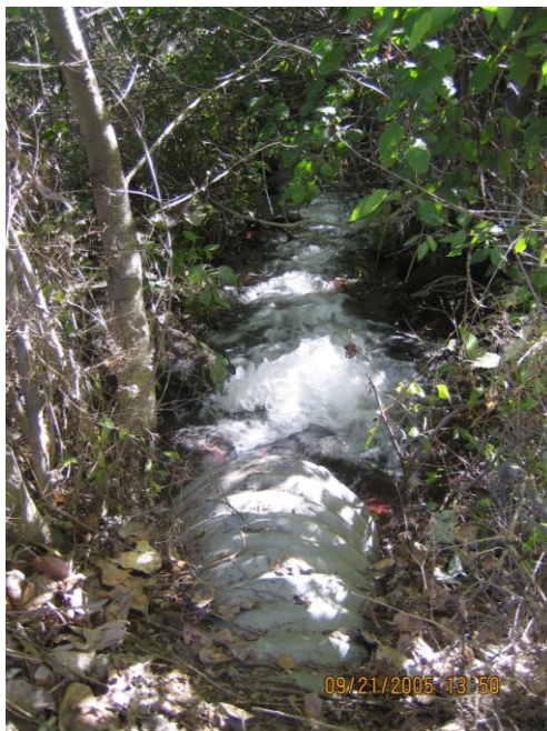
South Side – Looking South
