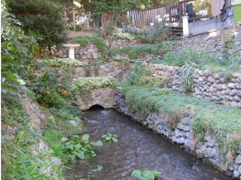
South Side – Looking South
