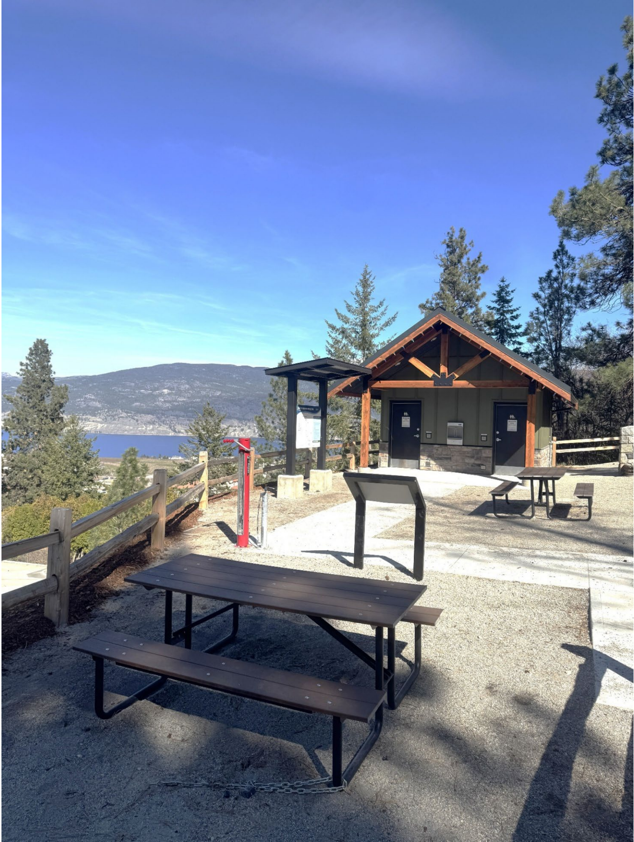
New Washroom Building Area
