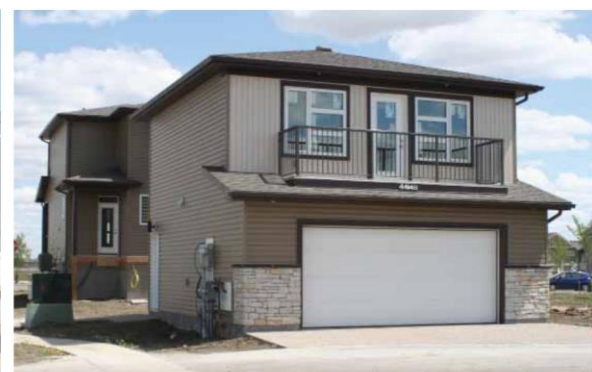
Laneway House Pilot Project in Harbour Landing, Regina
