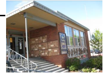
Mid - 20 th Century Modern Retrofit
