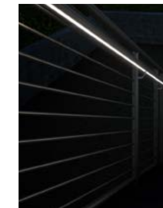
LED strip light embedded in railing
