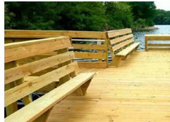
Seating embedded into wood railing
