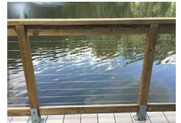
Wood railing with cable
