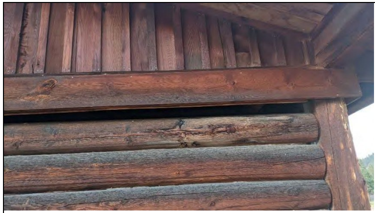
Figure 6 Gap between Infill logs and top of wall
