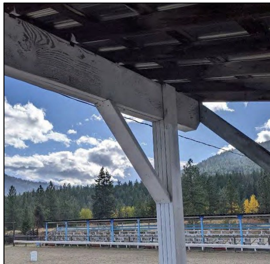
Figure 21 Front Knee Brace for Bleachers west elevation
