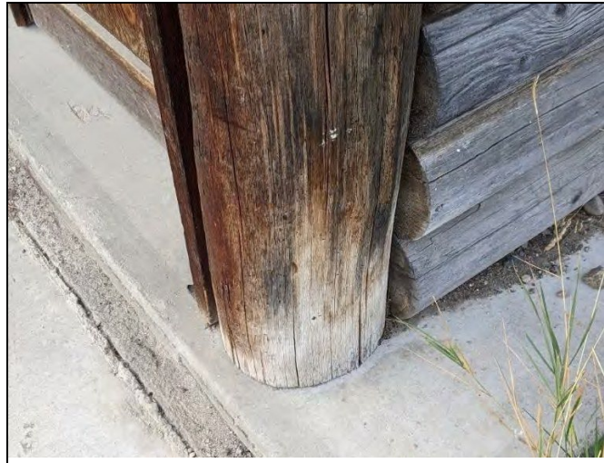
Figure 5 Moisture discoloration at base of posts
