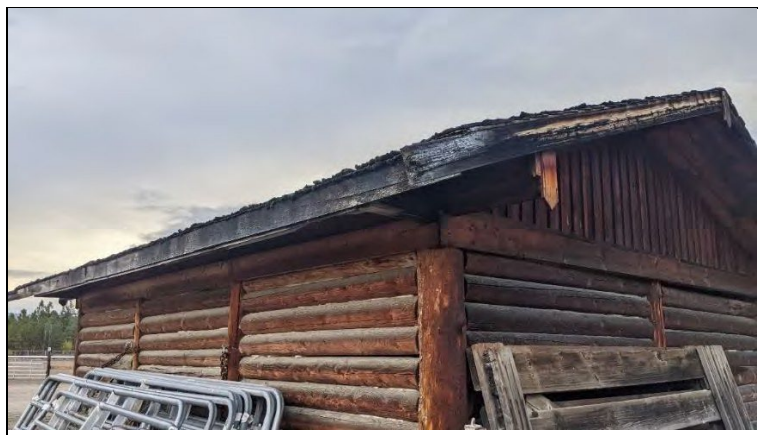
Figure 4 Wood Rot and Moss growth on Structure 1
