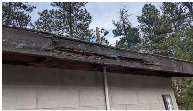
Figure 8 Damage to Eaves beam on Restroom east face
