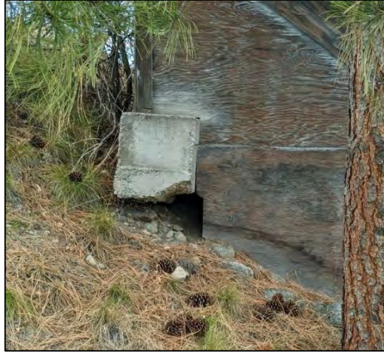
Figure 23 – Undermining of foundations at rear of bleachers
