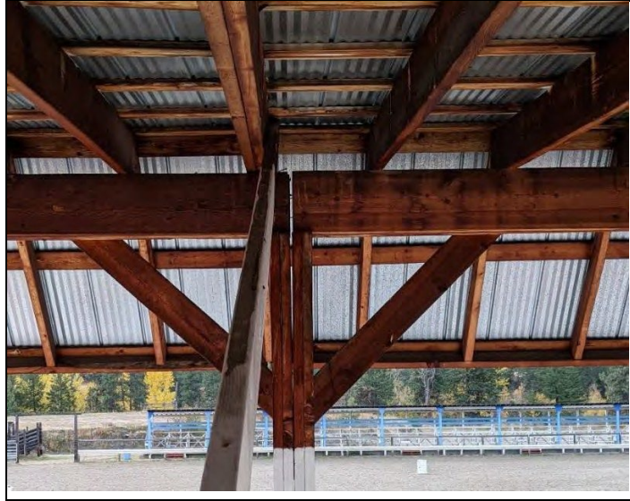
Figure 25 - Built up post opening up at top.
