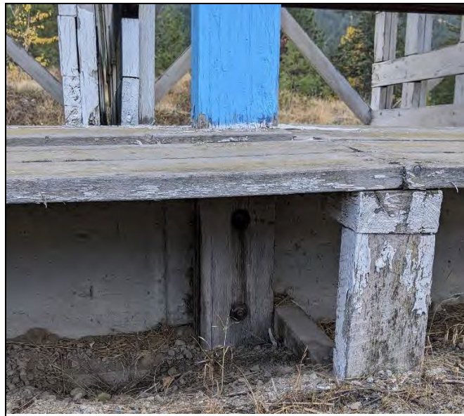
Figure 18 Post connection to concrete rising wall
