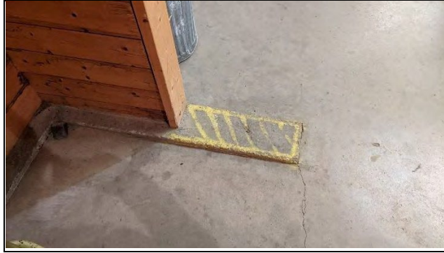
Figure 15 – Original extent of fin wall
