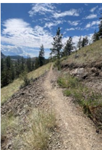
Failing Bench Cut
