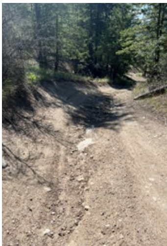
Tread Cupping, Berms & Erosion
