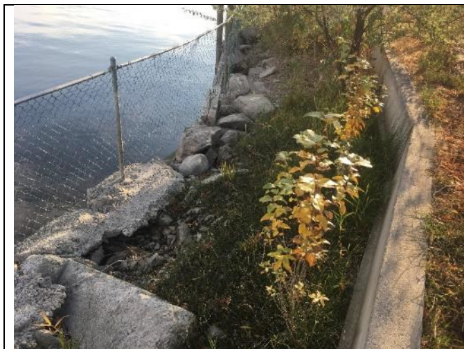
6-Old Timber Wall Retaining Material in Front of Concrete Wall – Concrete Wall has Exposed Footing
