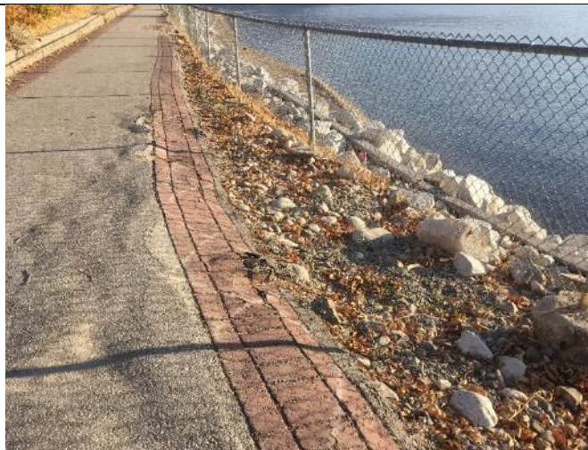
4- Submerged Path, Base Materials Mobilized Causing Uneven Asphalt Surface with Visible Erosion Damage
