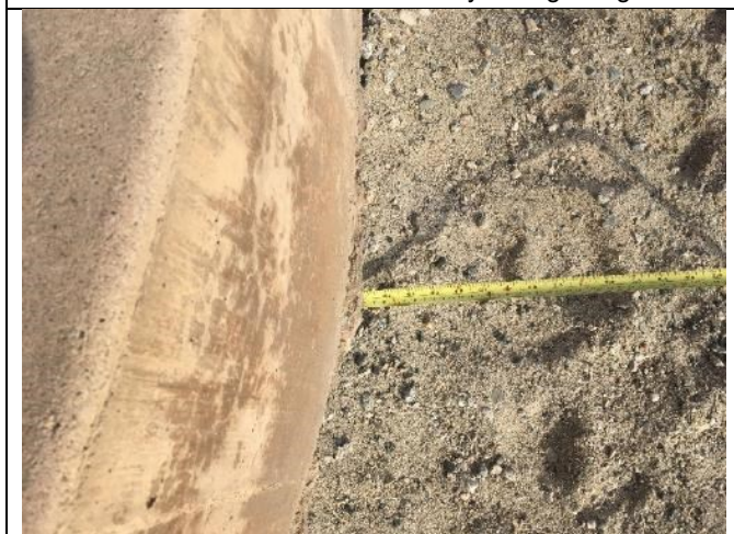
8a-Concrete Pathway is Undermined ~40"
