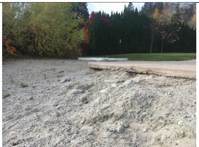
8a-Concrete Pathway is Undermined and Scouring
