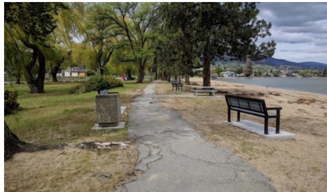
Photo: 9 Main park pathway is asphalt damaged by flooding and tree roots.
