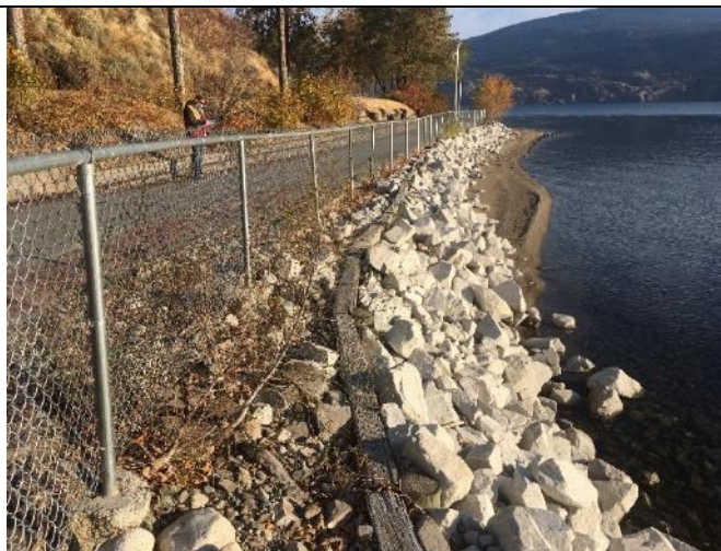
4-Emergency Riprap Placed along Wall is Steep with no Filter
