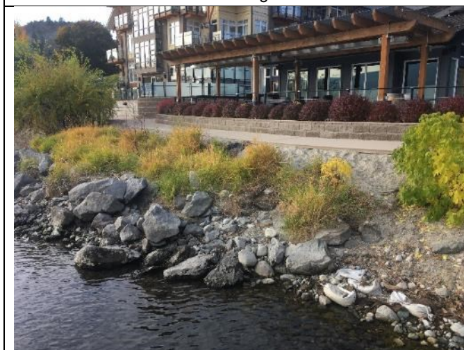
8b-Concrete Pathway is Undermined and Scouring
