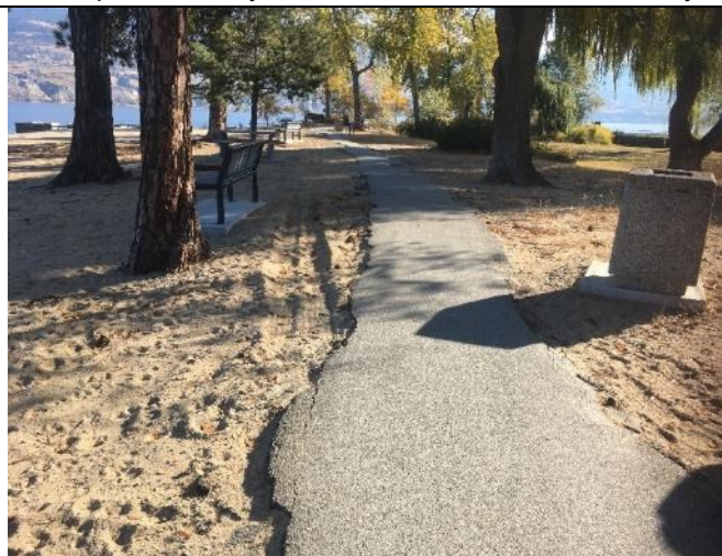
13-Asphalt Pathway has been Eroded and Damaged
