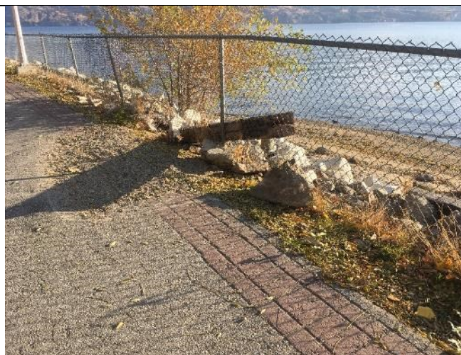
4- Pathway Susceptible to Erosion and Sediment Deposit where Old Timber Wall Sections are Damaged
