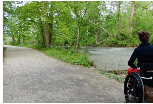
② Roadbase and limestone screening surfacing provides accessible pathway circulation.
