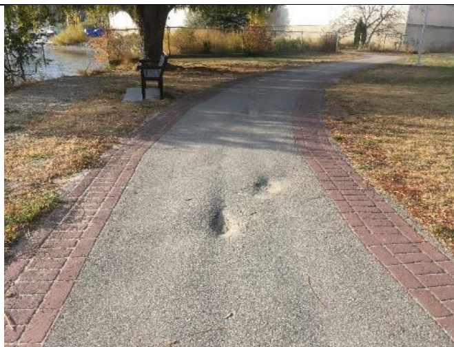
7-Sinkhole Developing in Center of Pathway
