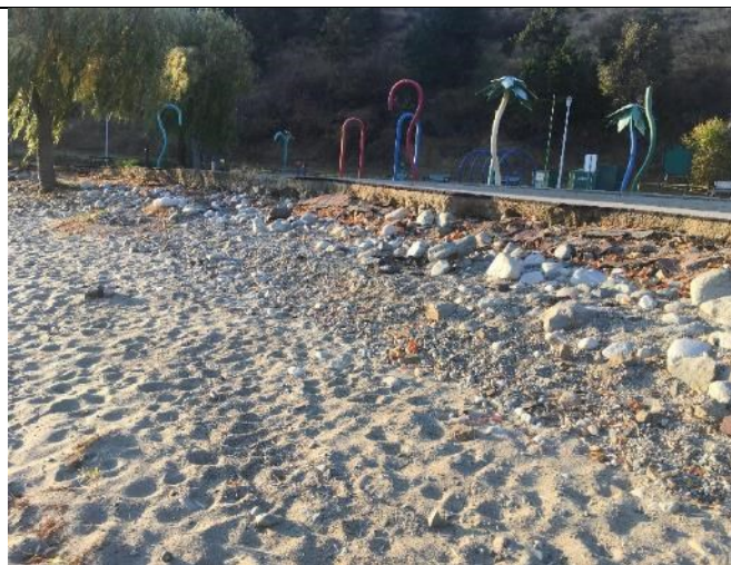
3-Pathway Adjacent to Waterpark Scouring along Eroding Beach
