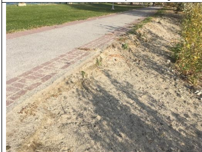
7-Erosion of Bank and Pathway is Beginning
