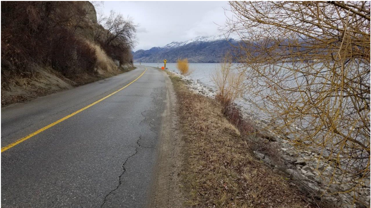
Photo 1.8: Segment #2 – Looking North – Asphalt and Road Structure Failure
