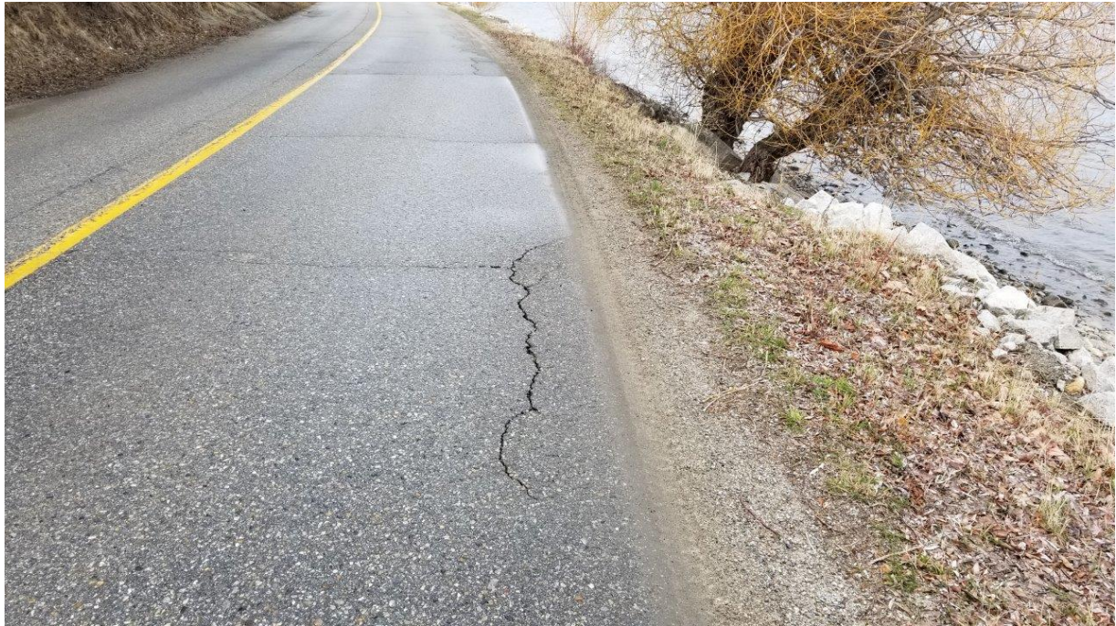
Photo 1.4: Segment #1 – Looking North – Asphalt and Road Structure Failure
