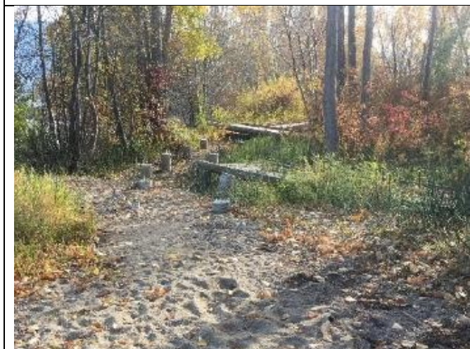
10-Boardwalk Section has been Uplifted and Displaced off Foundations
