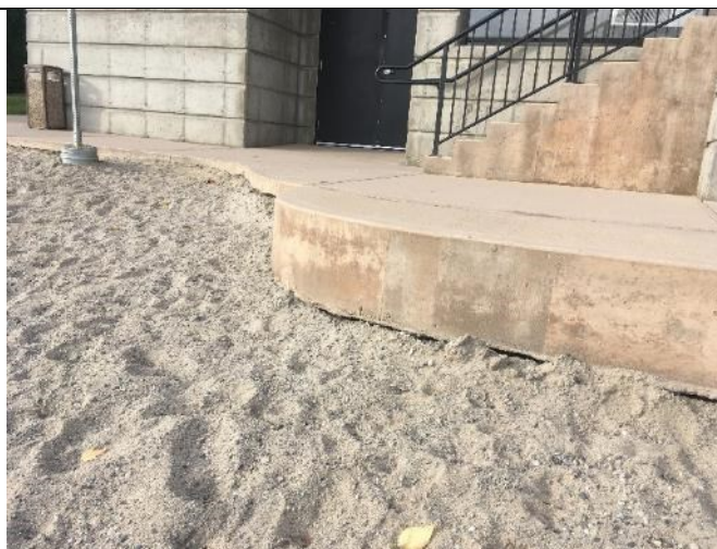
8a-Concrete Pathway is Undermined and Scouring
