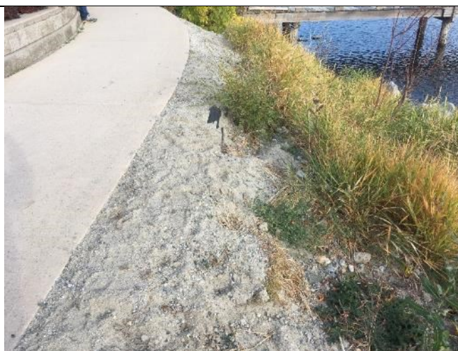
8b-Concrete Pathway is Susceptible to Scour and has Exposed Geotextile
