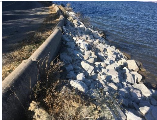
1-Barriers are Undermined along Eroded Bank
