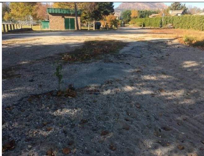
13-Asphalt Parking Lot has been Eroded
