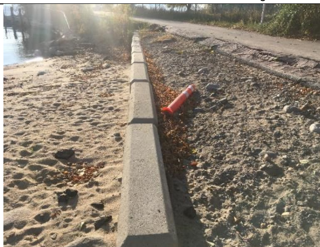
6-Lockblocks Retaining Material in Front of Pathway
