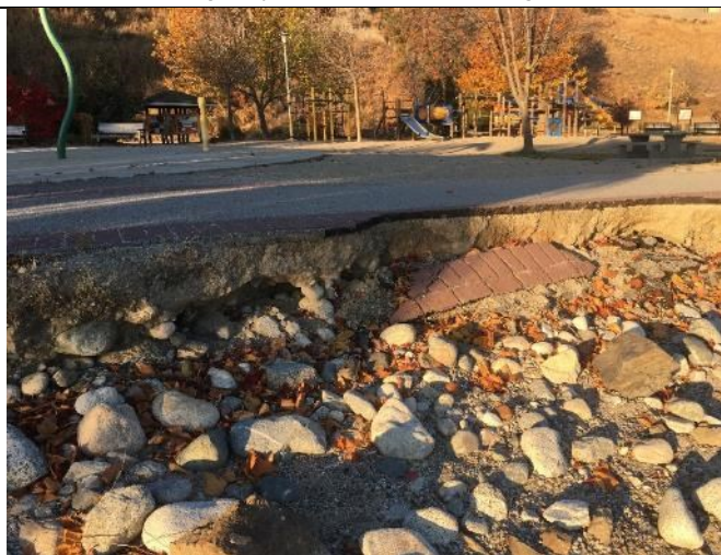
3-Sections are Undermined and Failing
