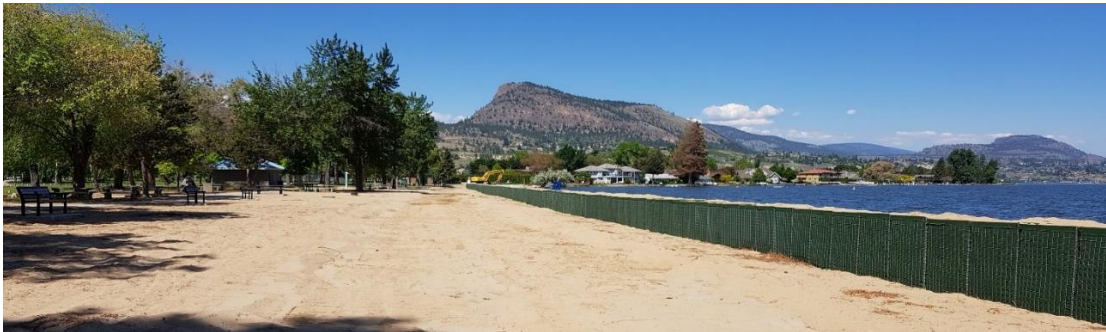
Photo: 10 Sand-filled gabions installed for temporary flood protection in 2018
