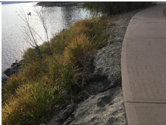
8b-Geotextile Retaining Material is Exposed and Damaged
