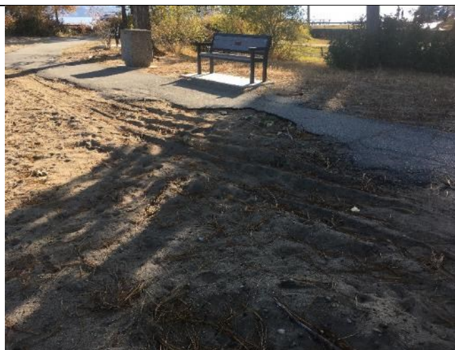
13- Asphalt Pathway has been Eroded and Washed Away
