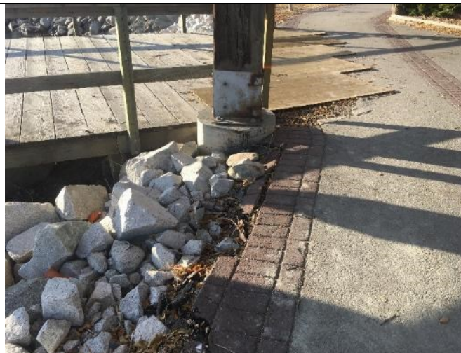
4- Pier Abutment Scour with Holes Boarded with Plywood
