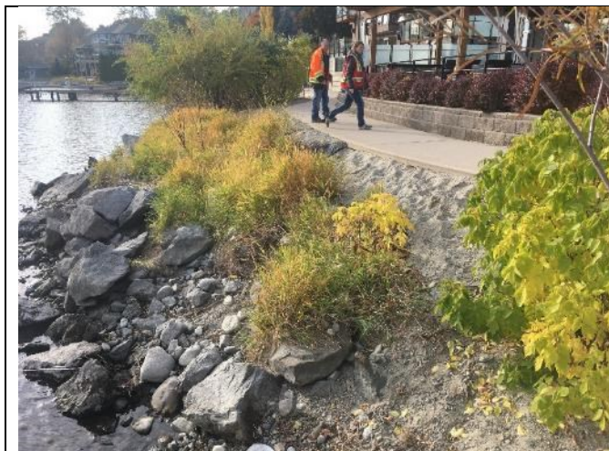
8b-Vegetated Point is Exposed to Waves and Actively Scouring
