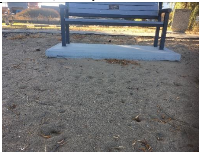
13-Undermined Bench Foundations
