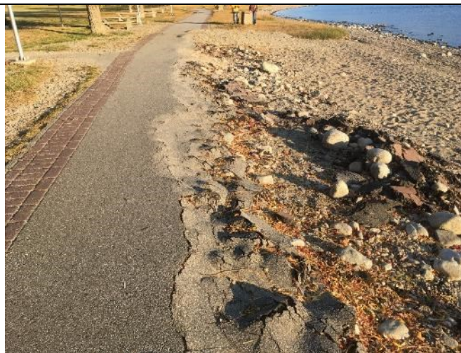
3- Section of Pathway along Beach is Eroding and Washing Away
