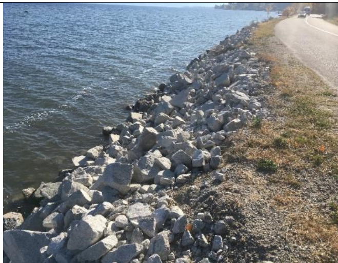
1-Emergency Riprap installed Along Bank
