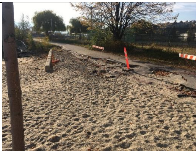
6-Significant Loss of Pathway from Erosion
