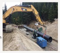
meet Dam Safety Regulations. Installation then began on the new 48-inch, high density polyethylene pipe (HDPE), and pouring concrete for the intake, outfall, and gate control structures. Geotextile fabric and rip rap were installed on the front face of the dam for erosion protection.
