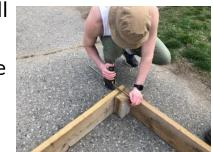
You will have the two sides (long pieces) left, the ends with the posts are now used to screw on the sides. You might need to use some wood clamps to help hold the frame together. Make sure your frame is square, finish off the frame with the center support, by using the saw and cutting to length the inside distance from the bed, side to side. Then screw the support in the middle of the bed to create a strong frame.
