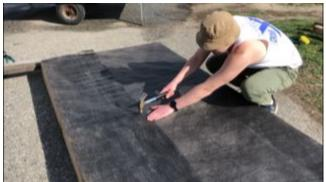
You are almost done building the garden bed. Using landscape fabric you can save time by not weeding as much. Pick which side of the frame you would prefer to be on the bottom, and then cut the fabric with scissors to the size of the frame. Use nails or staples to attach the fabric to the bottom of the bed.
