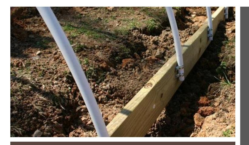
Next You are going to attach pcp pipe connecting on both sides so you can put on the plastic tarp you can attach it using clamps or what I did just stick both sides into the ground
