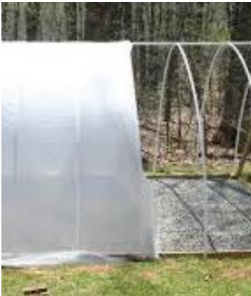
For this step you are going to want to get plastic tarp that goes around the the whole area so that it all seals and there are no gaps and to actually attach it you are going to need to pull the plastic down to the wood base and then get a wood strip and nail the wood piece to the other wood piece trapping the plastic wrap and making it tight you will want to do it on all sides
