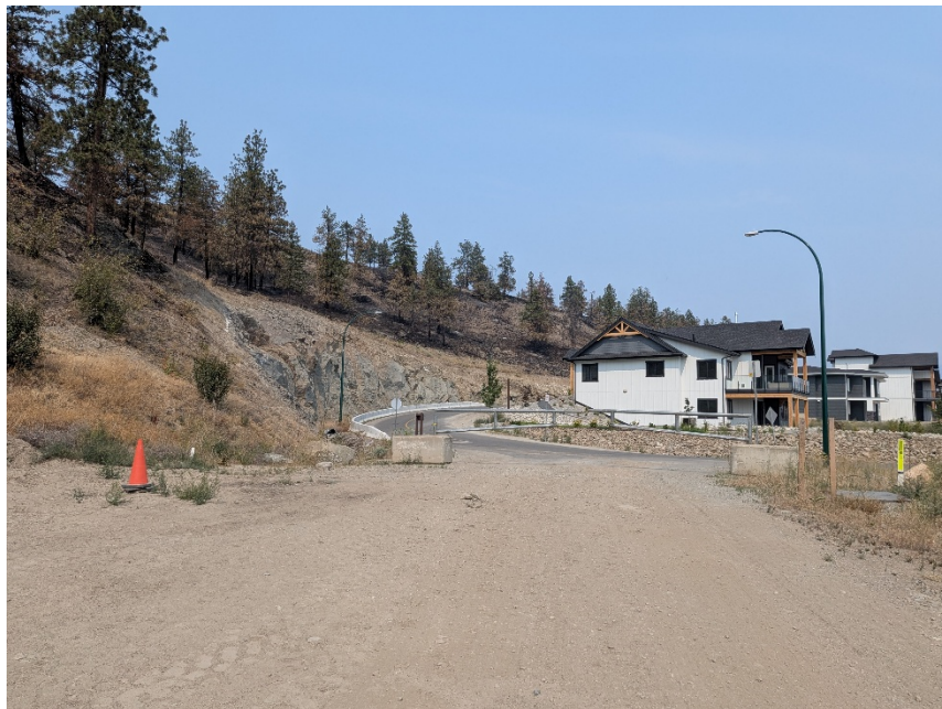
Photo 4. Slope above Dickinson Place, looking north.
