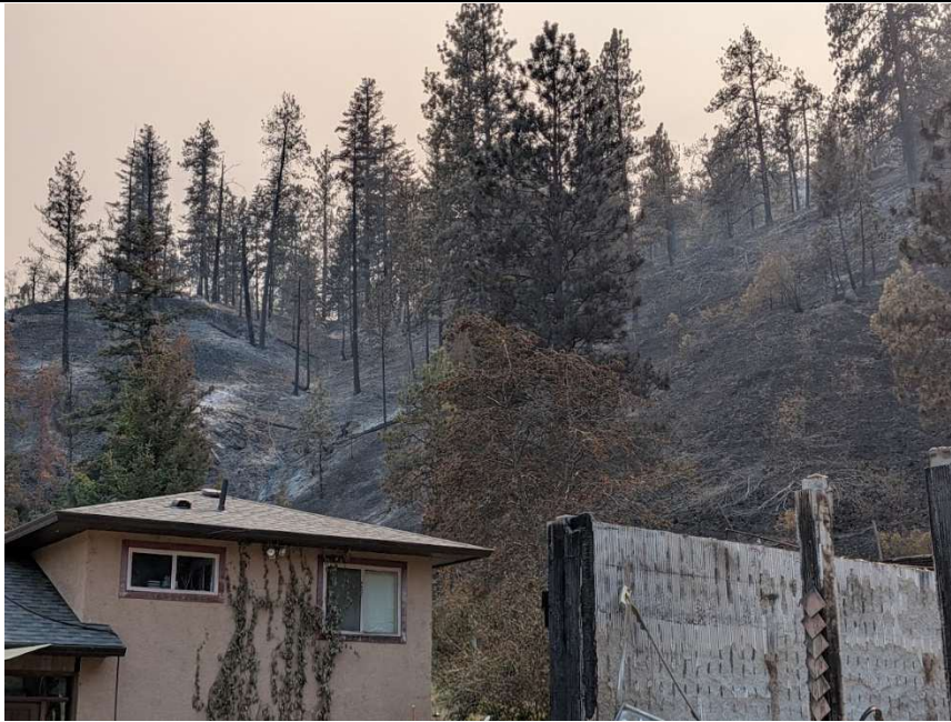
Photo 5. Burned gully immediately upslope of remaining house on 16218 Garnet Valley Rd.
