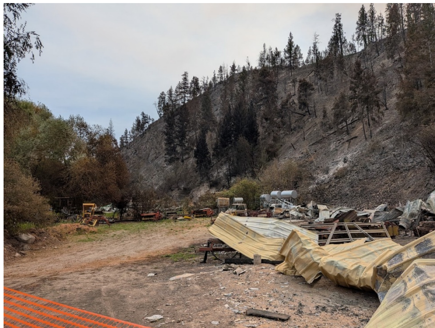
Photo 4. Heavily burned steep slope above 27006 Garnet Valley Rd looking south.
