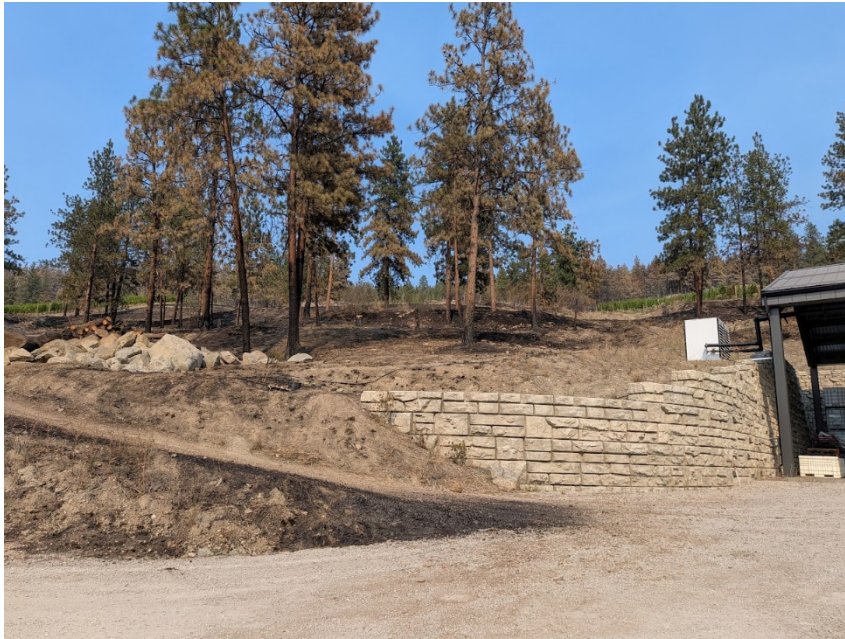
Photo 1. Burnt slope and gully above the crush pad on 25205 Wildhorse Rd looking east.
