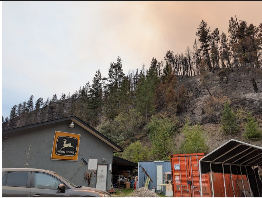
Photo 3. Burned slopes uphill of remaining buildings looking southwest.
