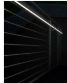
LED strip light embedded in railing
