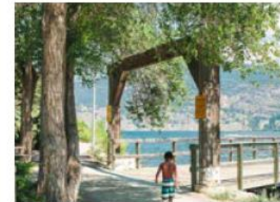
Existing entrance archway
