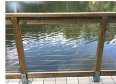
Wood railing with cable
