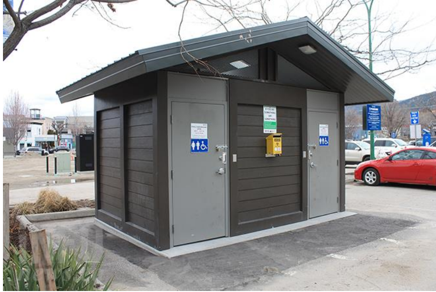
Figure 47: Washroom facility in Penticton
