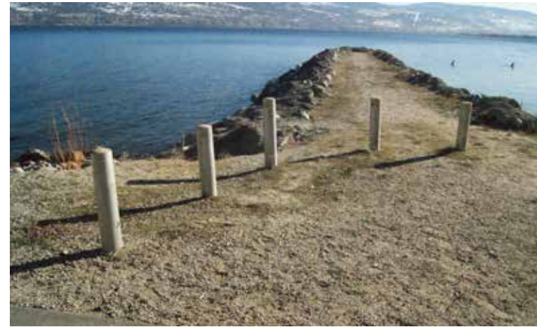
Breakwater and bollards
