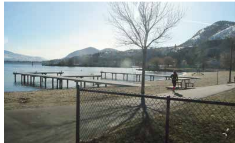
View South toward F and I docks and beach
