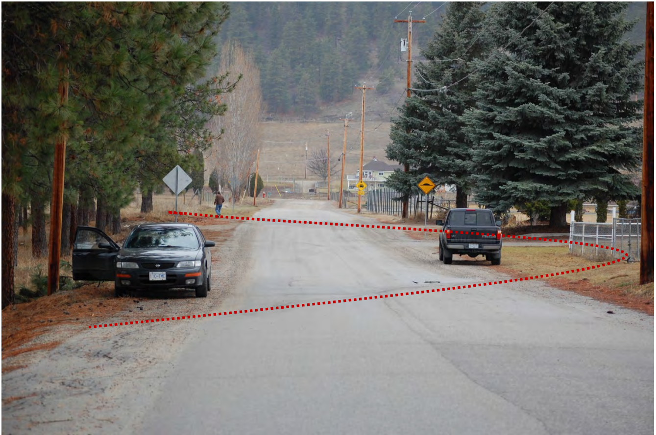
Photograph 3801: Looking west along abrupt roadway depression (dip) that extends across both lanes and to about 5 m into the north property at 10920 Canyon View Road.
