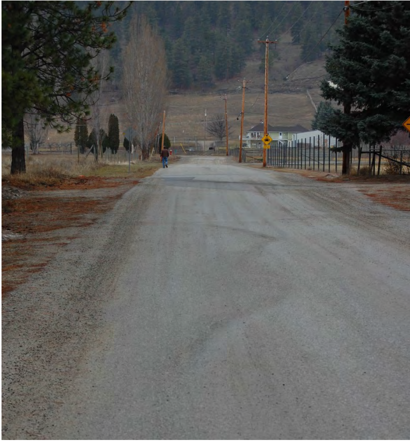
Photograph 3809: Looking west along Canyon View Road at inside crescent shaped crack that extends to about the roadway centre line. This feature has developed within the past year or so. The crack feature is about 25 m in length and has an abrupt drop of about 50 mm.
