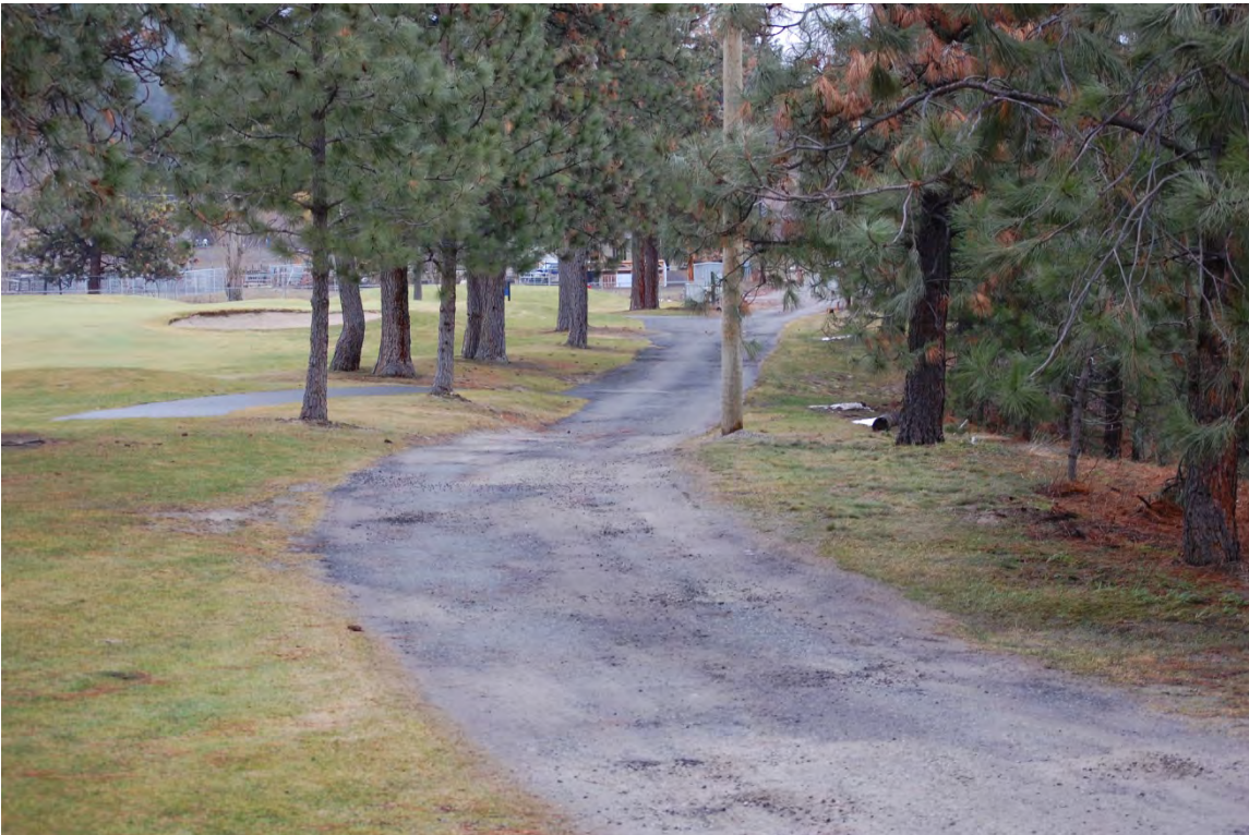
Photograph 3864: Looking north at localized depression along section of access road to the golf course maintenance yard. Piezometer/monument P1 is located about 10 m north of the narrow golf pathway (hidden behind larger trees) that runs to the left on the photograph.
