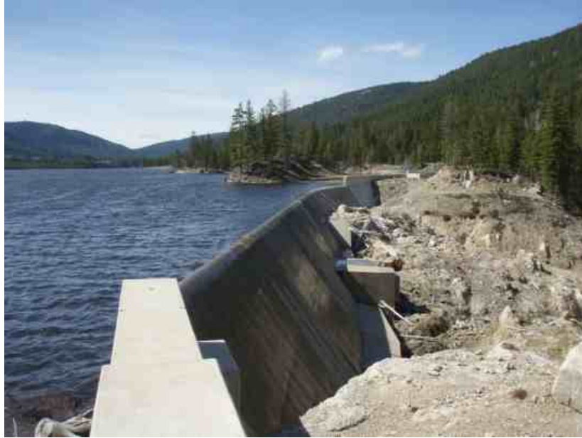
Photo 1 Spillway – Viewed from the East
