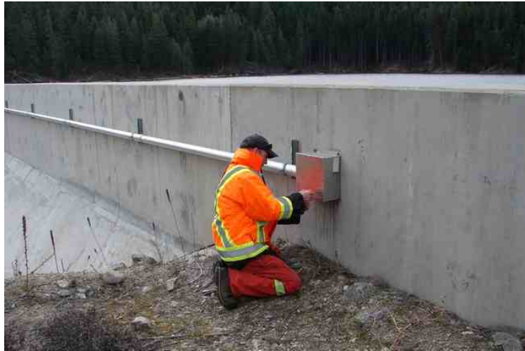
Photo 4 Piezometer Monitoring Station – Spillway Left Abutment
