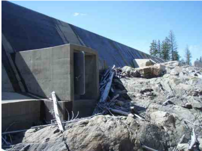
Photo 2 Spillway Gallery - Entrance
