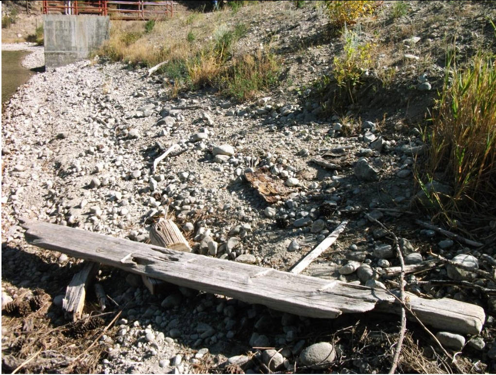
Photo 3 – View of upstream slope, above waterline, showing beaching on slope, Gate Tower in background.
