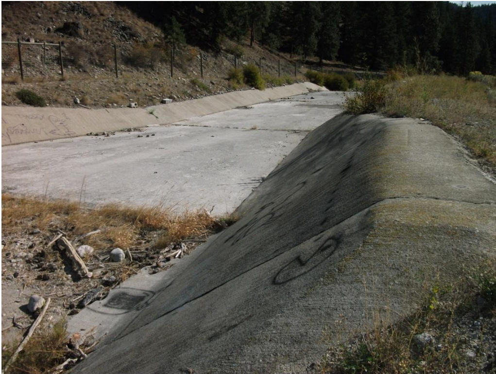
Photo 12 – View looking downstream showing concrete spillway sill and channel lining.
