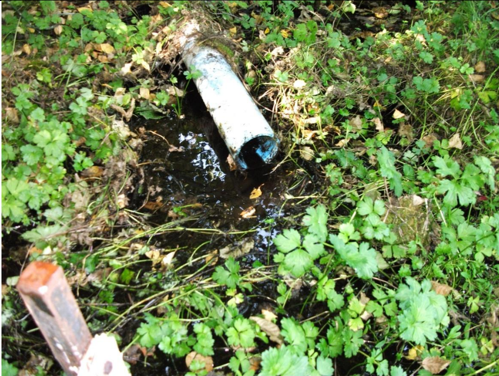
Photo 7 – View looking at right side of creek bank, showing six inch diameter drain pipe outlet.
