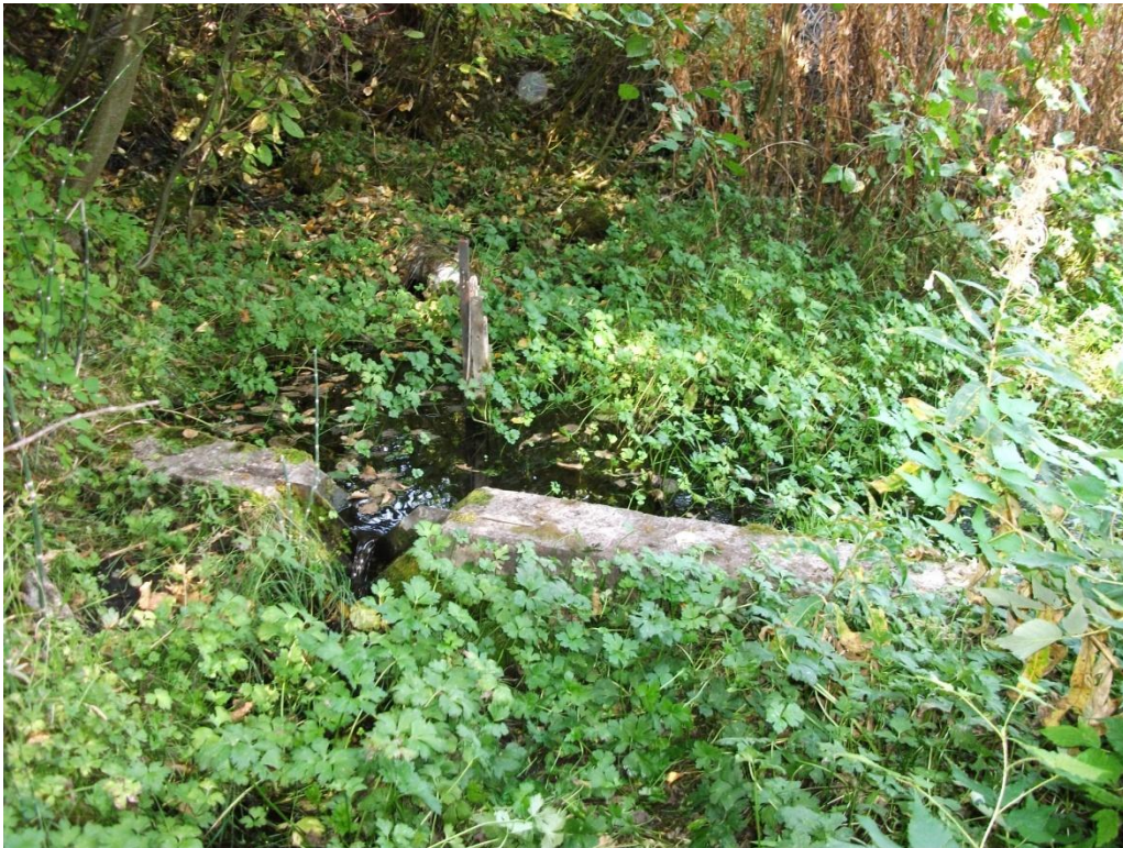
Photo 6 –View looking upstream showing V-notch weir in toe seepage collection works. A six inch diameter drain pipe outlet is situated in the background.
