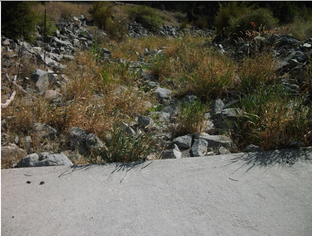
Photo 13 – View looking downstream showing spillway rip rap channel.
