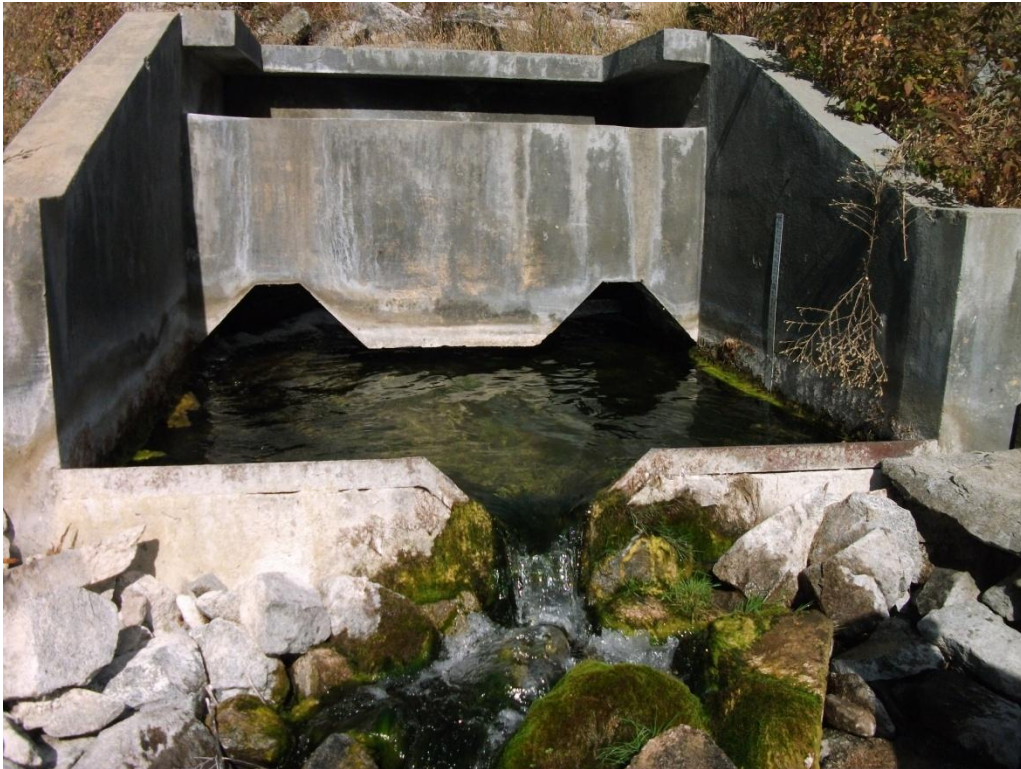
Photo 4 – View looking upstream showing outlet stilling basin. Note water release for fish purposes (fish gate).
