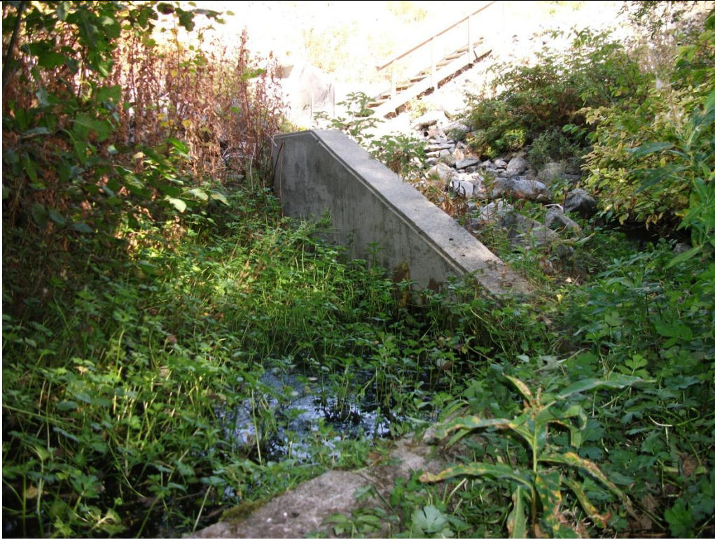
Photo 5 – View looking upstream showing concrete wall for toe seepage collection works in foreground; outlet stilling basin, timber stairs in background.
