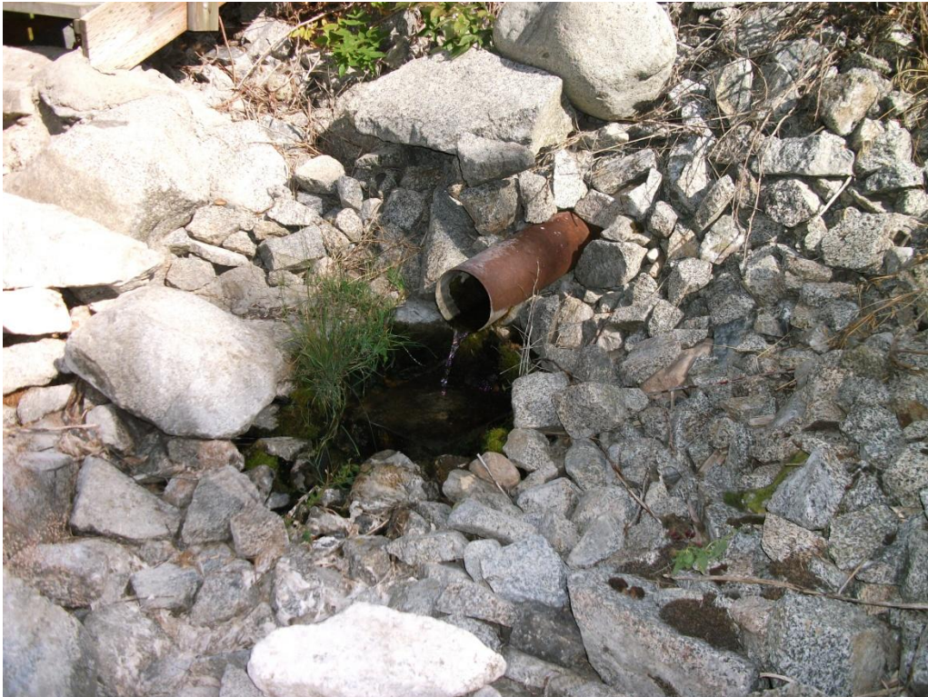
Photo 8 – View looking at left side of creek bank below outlet, showing six inch diameter drain pipe outlet, near timber stairs.
