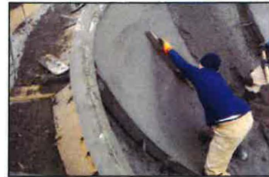
Ecosmart Concrete over crushed recycled concrete sub base
