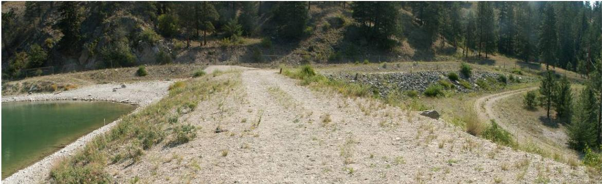
The Garnett Reservoir full-pool water elevation is approximately 632.76 metres with a total water surface area of 38.3 ha. Garnett Reservoir is annually filled by a sub-catchment area of approximately 9,100 ha (91 km<sup>2</sup>). With a total live storage volume of 2,360 ML, Garnett Reservoir comprises about 14% of the total District of Summerland reservoir storage capacity.
