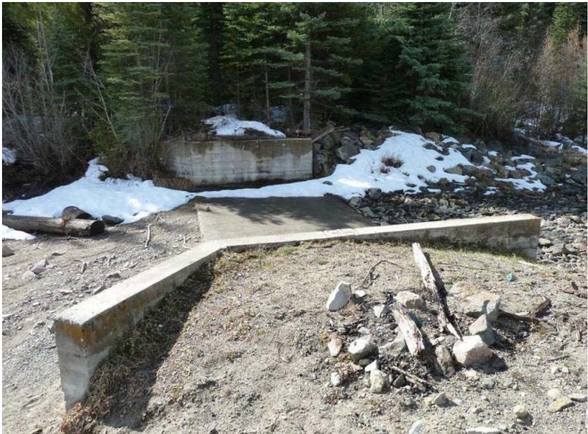
Figure A1.4 - Headwaters No.1 Reservoir Spillway
