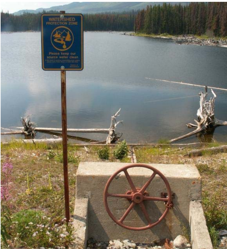
Figure A4.4 – Headwaters No. 4 Dam - Gate Control
