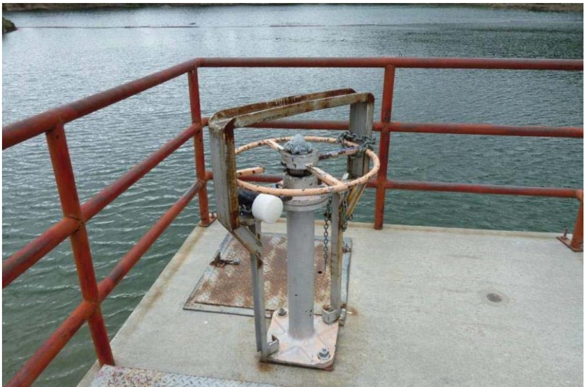
Figure A11.4 – Garnett Dam Gate Control
