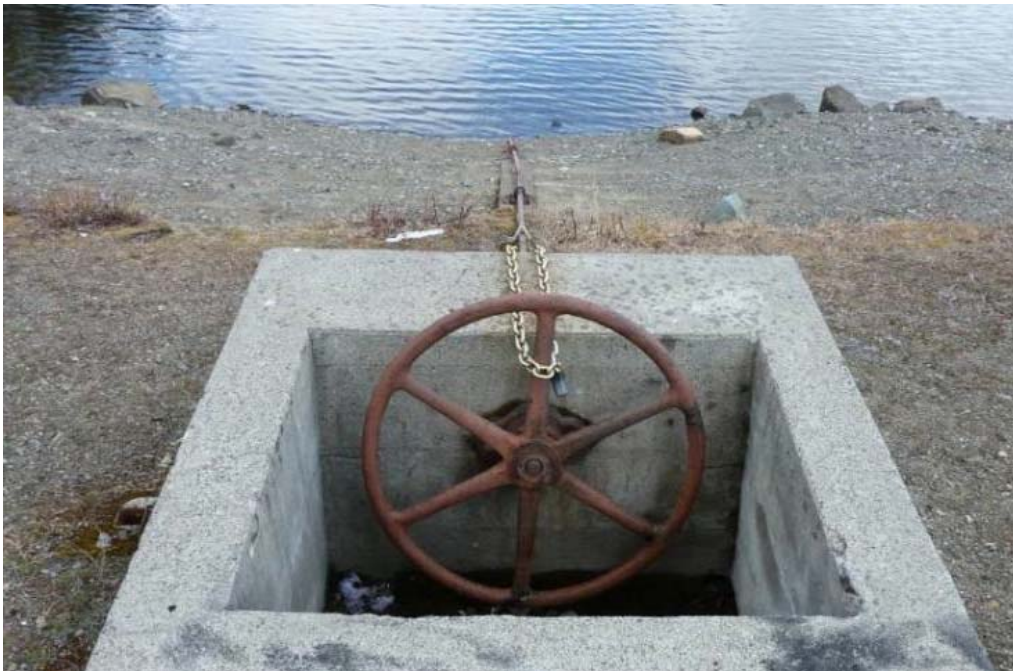
Figure A3.4 – Headwaters No. 3 Dam - Gate Control
