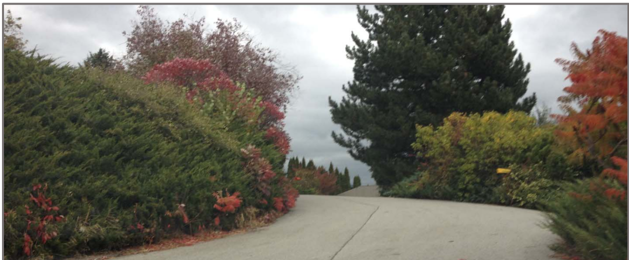
Figure 3: Horizontal Curve and Landscaping on Latimer Ave Constrain Sight Lines
