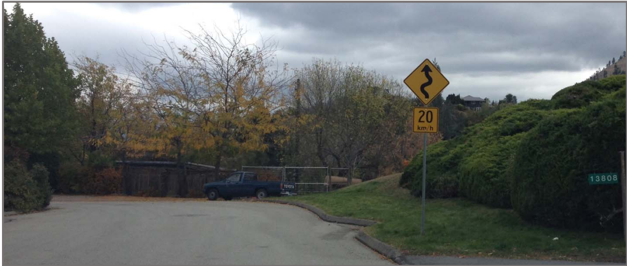
Figure 2: Curve Warning with 20 km/h Advisory Speed Entering Horizontal Curve on Latimer Ave
